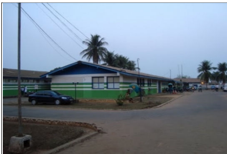
Figura – 1 Hospital Regional de Ariquemes
