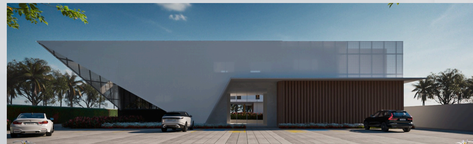
PLAYGROUND - FACHADA DE TRÁS
